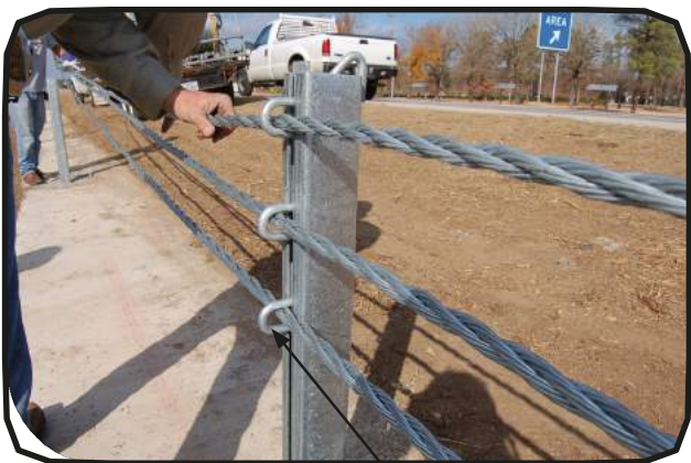
Installed Hairpin and Lockplate
